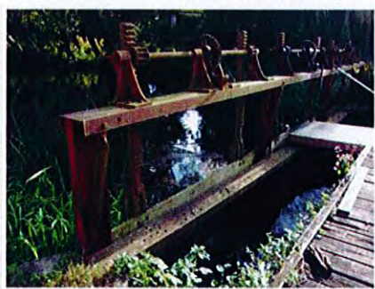
Fiskgaller, 67 graders lutning, spaltbredd ca 14–17 mm
