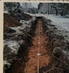
Figure 2: Installation of the electric cables and electrodes of monitoring system
